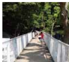
The south entrance to the Uribo Road
